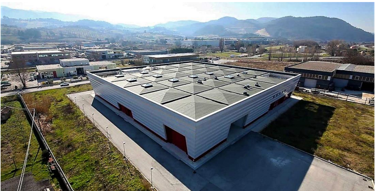
Santo Chiodo depot, external view (Spoleto, Italy) © ABAP Superintendency of Umbria
