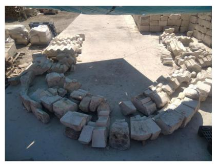
The Gothic arch reassembled at the St. Scholastica site with a view to its relocation © MiC
