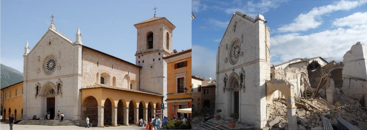
*Left: The Basilica of San Benedetto in Norcia before and after the seism of 30 October 2016; right: the rubble masonry literally crumbled, leaving inside the Basilica a four meters high rubble front © MiC*
